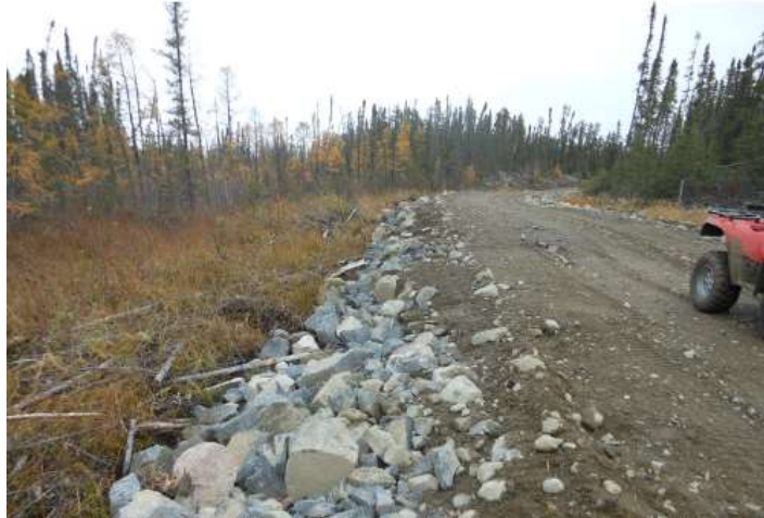
Figure 3. Angular aggregate may be used as permeable fill to facilitate wetland water movement.
