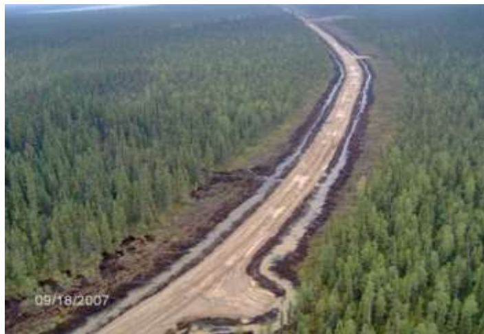
Figure 1. A resource road under construction across a conifer swamp.
