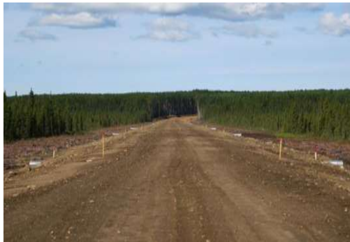
Figure 2. A resource road under construction with multiple culverts.
