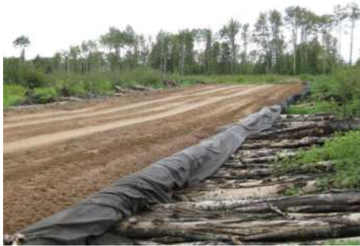
Figure 4. Corduroy installed to provide for water passage through a road.
