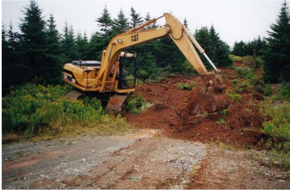
Figure 2. Forest road construction by excavator
