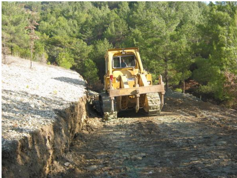
Figure 1. Forest road construction by bulldozer
